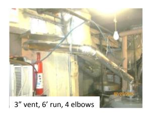
WI\_01 had a large opening downstream of the water heater (unused, partially repaired connection for a furnace)
