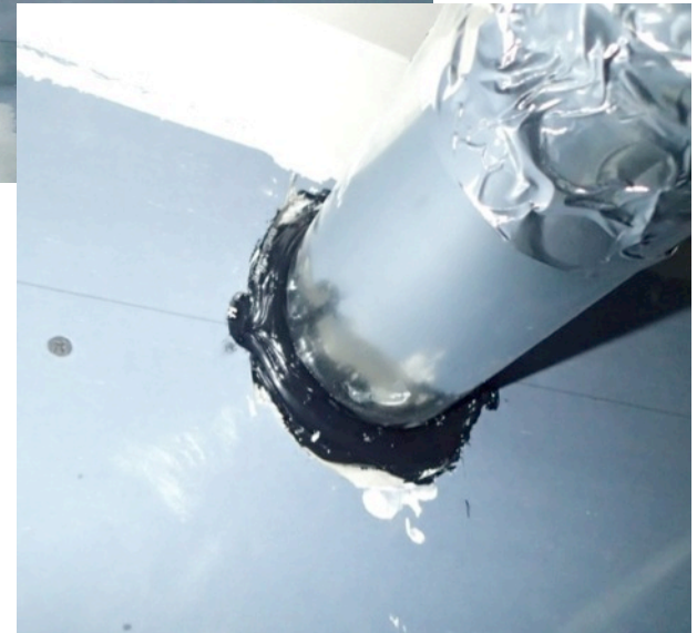
Duct – narrow enough to leave?
