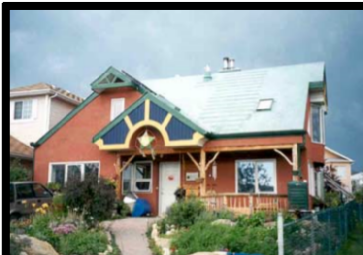
Fig. 1: View from S.W.
