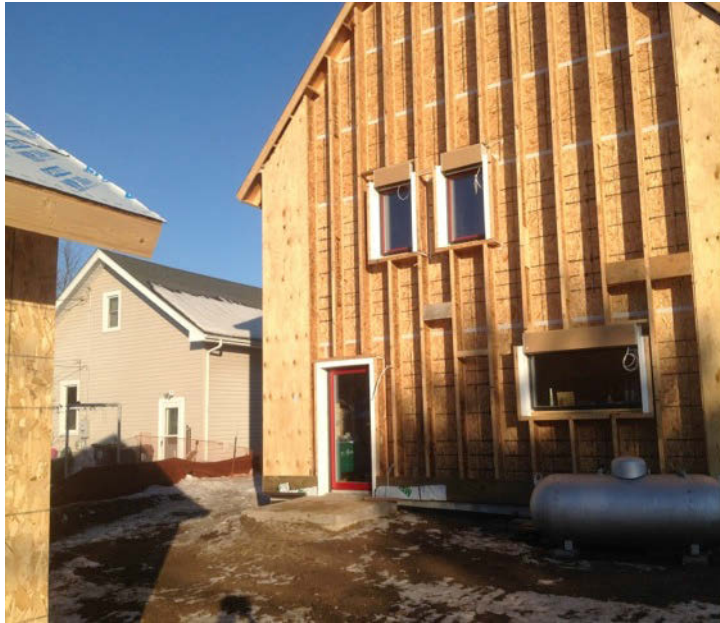
14" I-joist balloon frame
