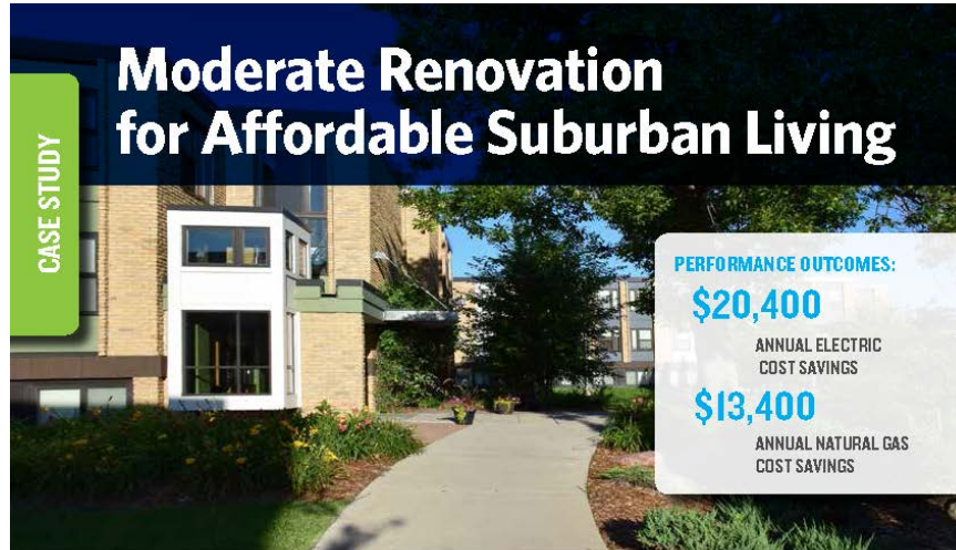
SIENNA GREEN I, NONPROFIT APARTMENT BUILDING, ROSEVILLE, MINNESOTA
