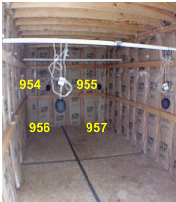
Roofpond (RP) Interior
