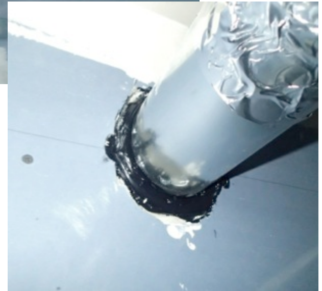
Duct – narrow enough to leave?
