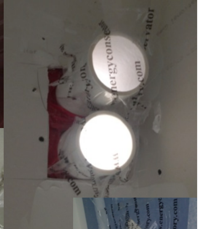
Combustion vents
