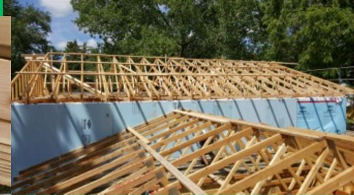
Foam board on house wall before roof truss
