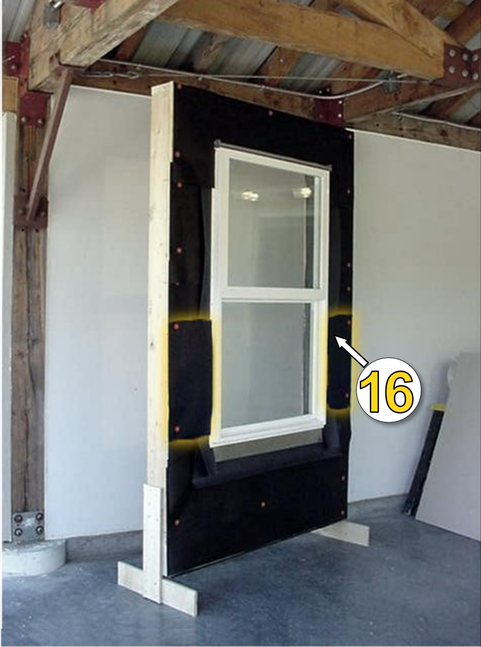
16 Building paper installation second layer third row (stager laps).
