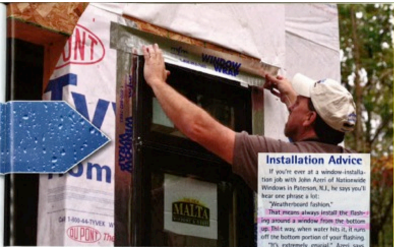
Proper installation of flashing around a window opening is crucial to prevent water infiltration.
