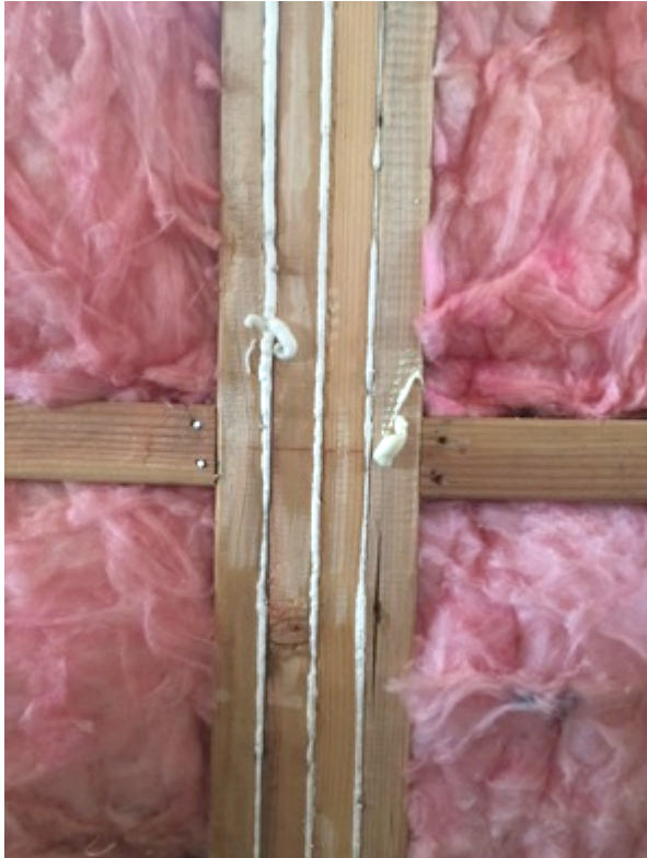
Can foam at seams where wood is joined
