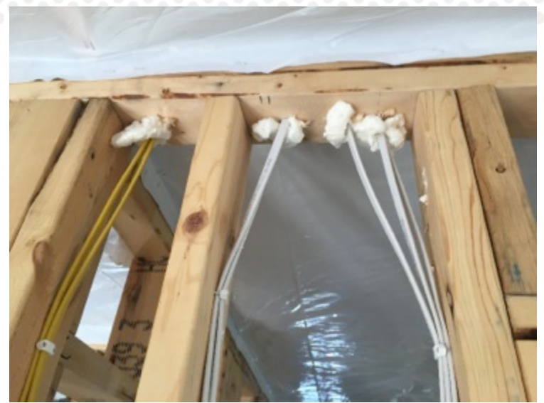
Can foam at wire penetrations
