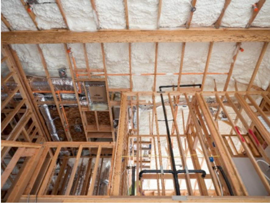
Foam at roof deck
