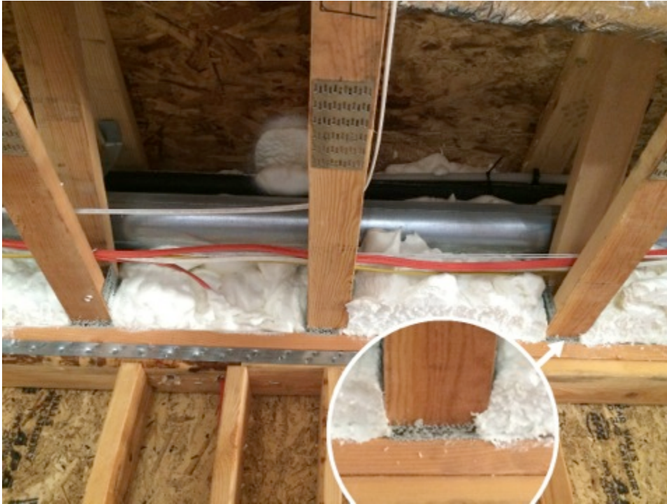
Seals formed under trusses
