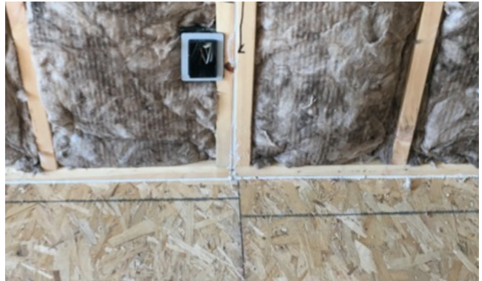
Caulk at sill plate
