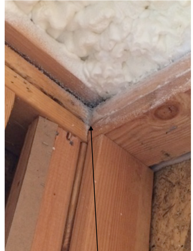
Seal formed at corner of wall assembly
