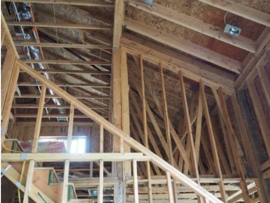
Exposed roof deck
