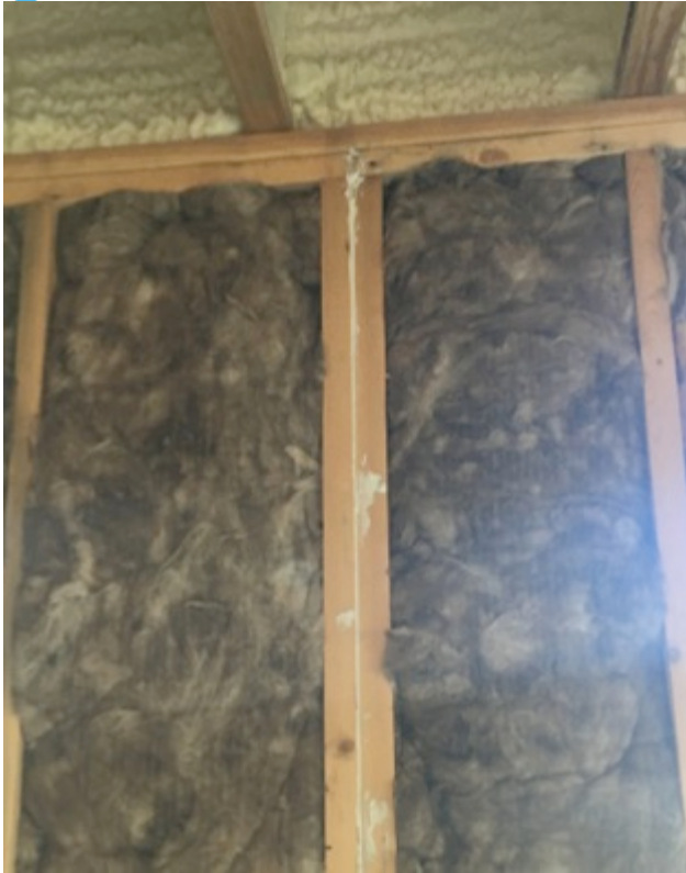
Caulk at seams where wood is joined
