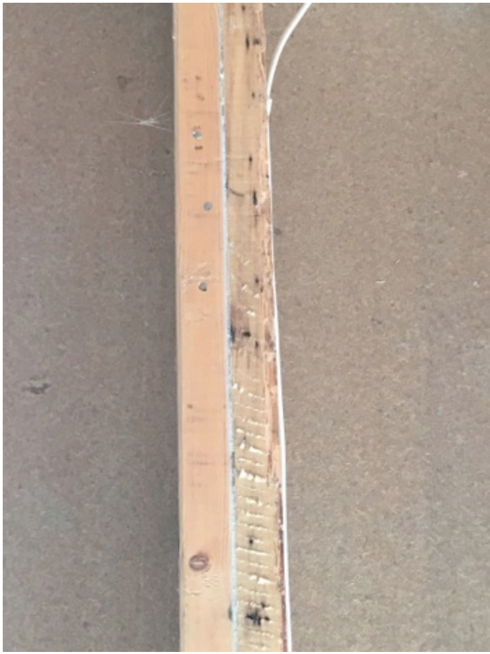
Seal formed between studs
