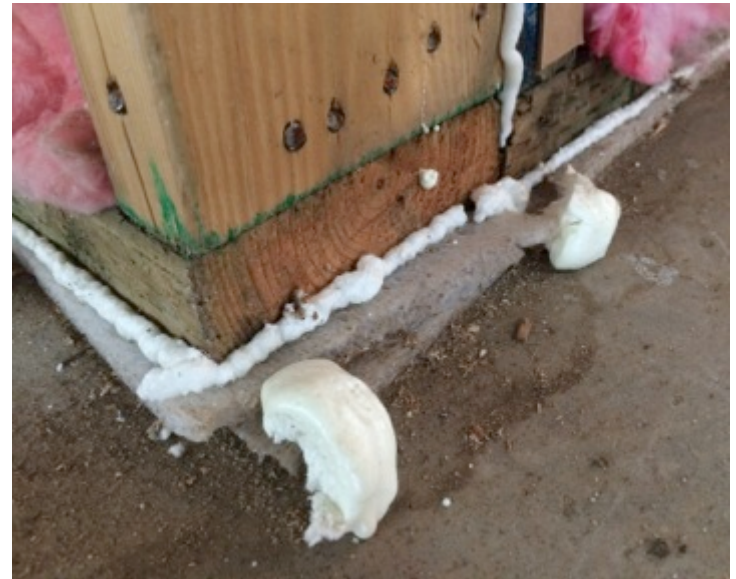
Can foam and gasket at sill plate
