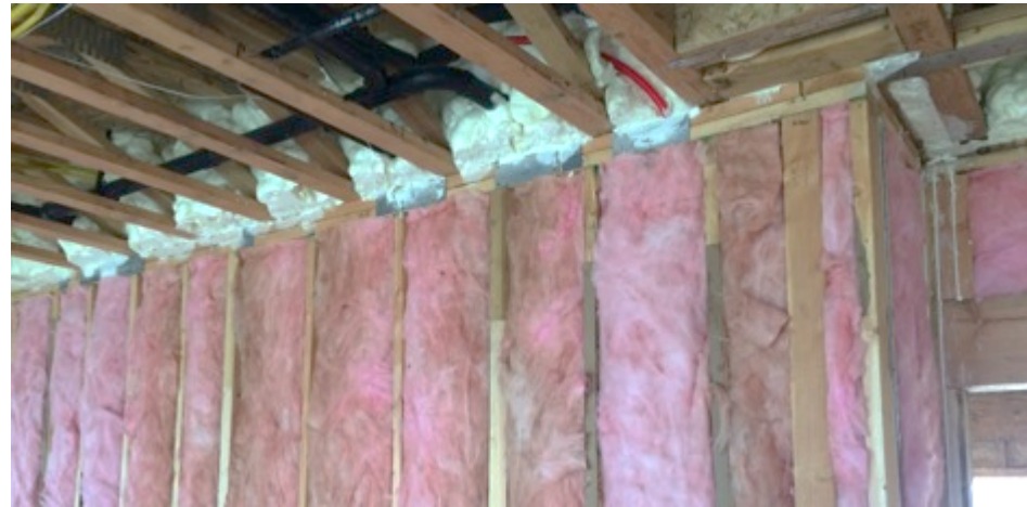
Foam at rim joist
