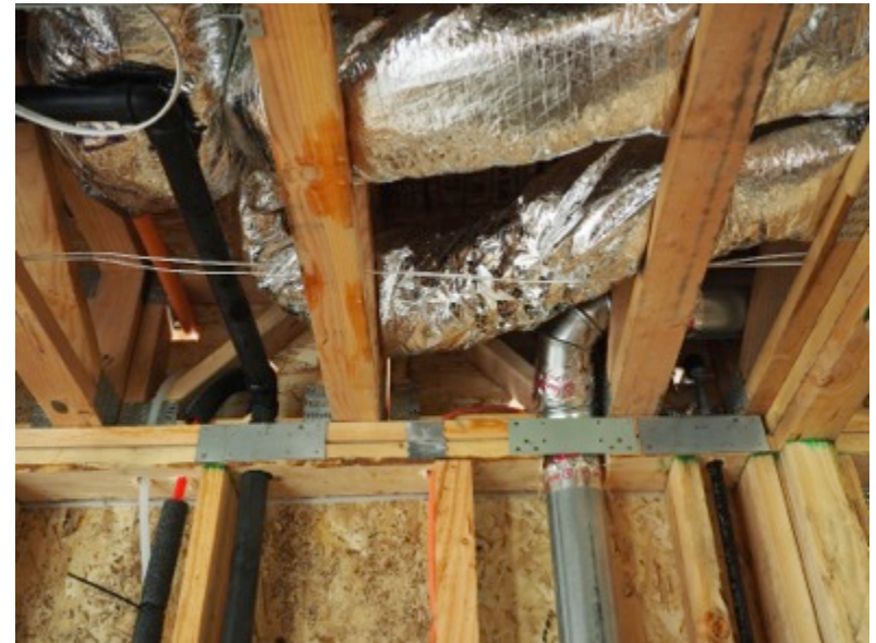
Rim joist penetrations
