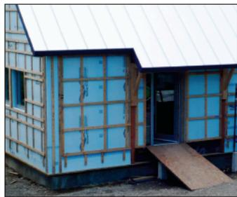
Unaware of the recently reported GWP implications of certain foam insulation materials, builder Todd Benson specified four inches of extruded polystyrene over 2x6 studs insulated with dense-pack cellulose in this net-zero-energy home.
