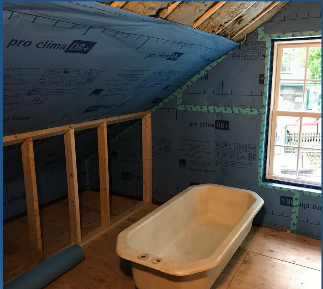
*Installation of Pro Clima variable-permeable vapor retarder in a bathroom over mineral wool batts - photo: Alex Wilson*
