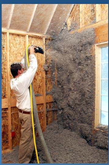
Damp-spray cellulose installation - photos: EnerSol
