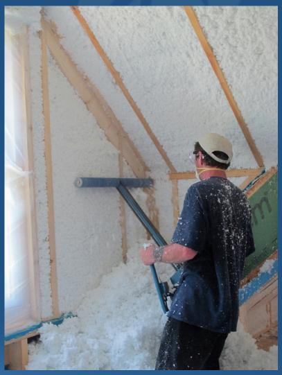
Cavity-fill: spray fiberglass (Johns Manville Spider) - photos: Alex Wilson
