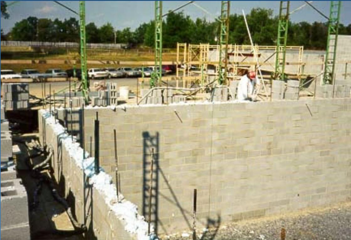
*Cementitious foam filling masonry cavities
