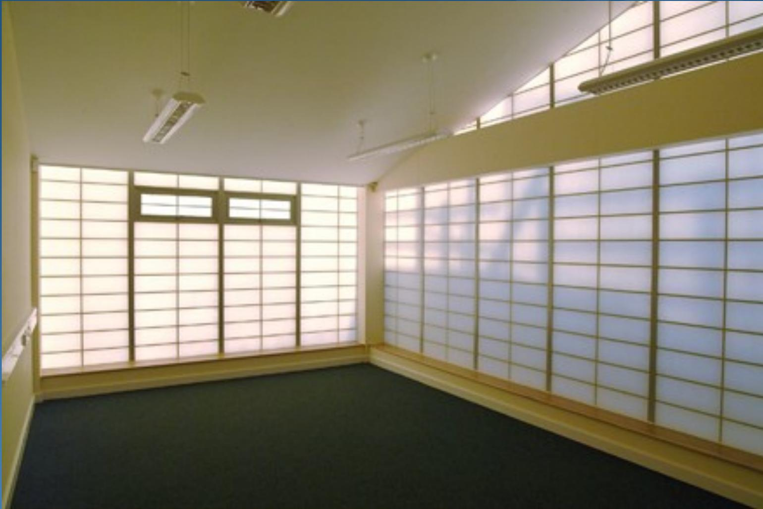
*Translucent glazing panels insulated with silica aerogel – photo: Cabot Corp.*
