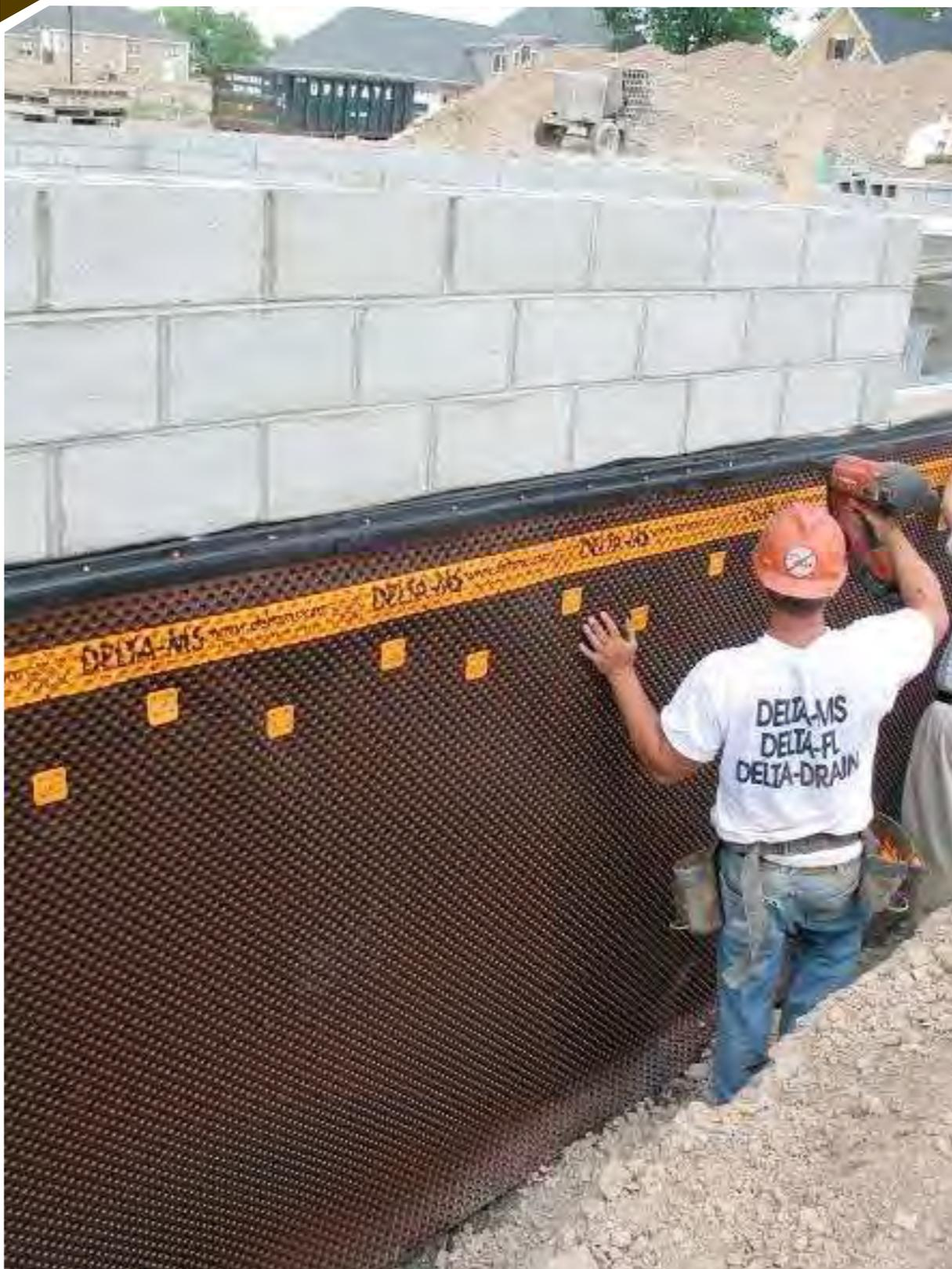
DELTA-DRAIN TO BE INSTALLED IN ROWS FROM BOTTOM TO TOP OF WALL, OVERLAPPING SHINGLE-STYLE
