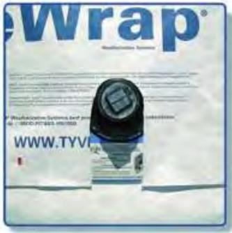
Step 2) Place 2nd layer of building paper over top of panel to bottom front edge or further down. Cut paper around protrusion. Now, ready for your choice of exterior finishes.
