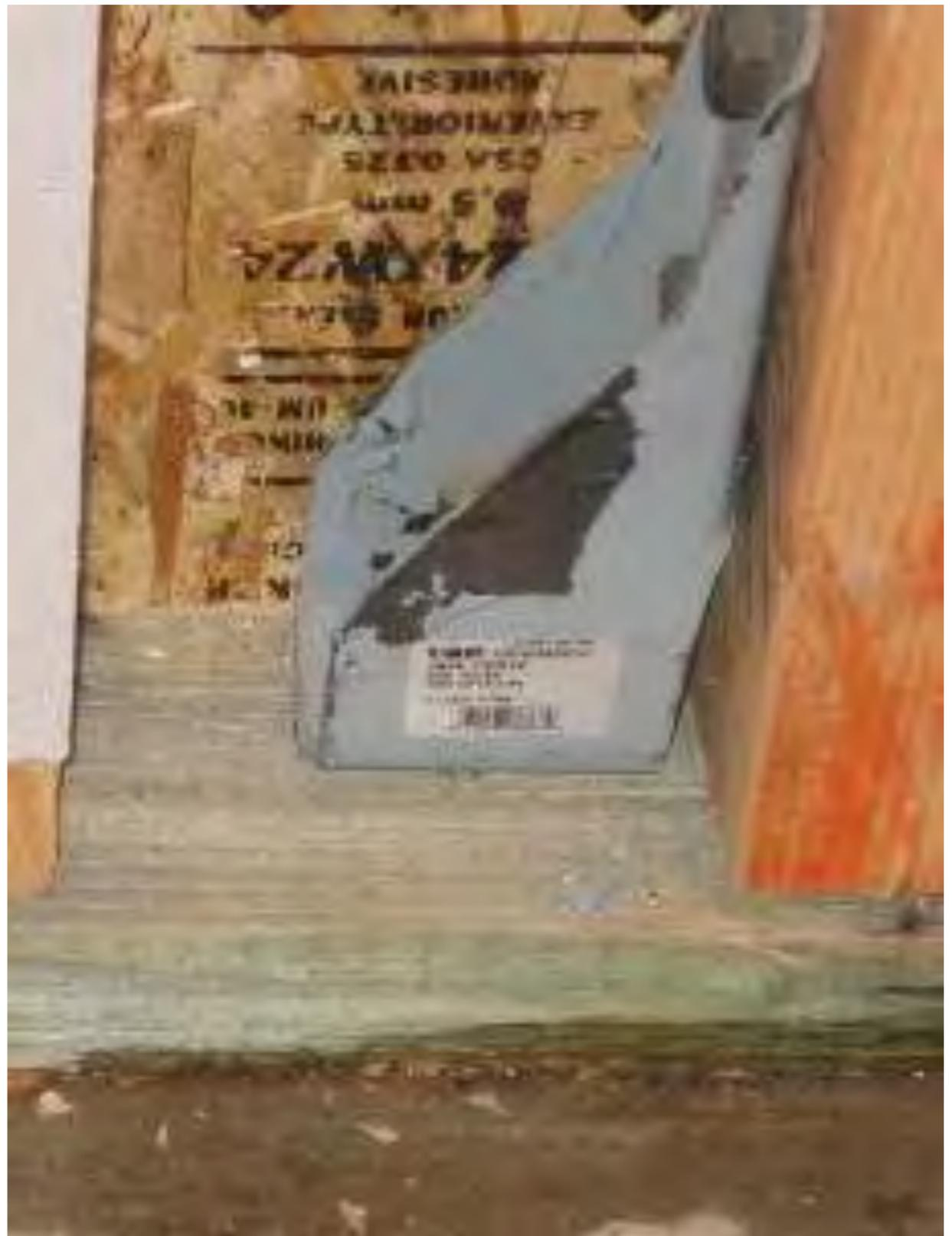
We often under invest in managing moisture. 80% of building failures=water related...yet less than 1% of total construction cost spent on managing water -flashings
