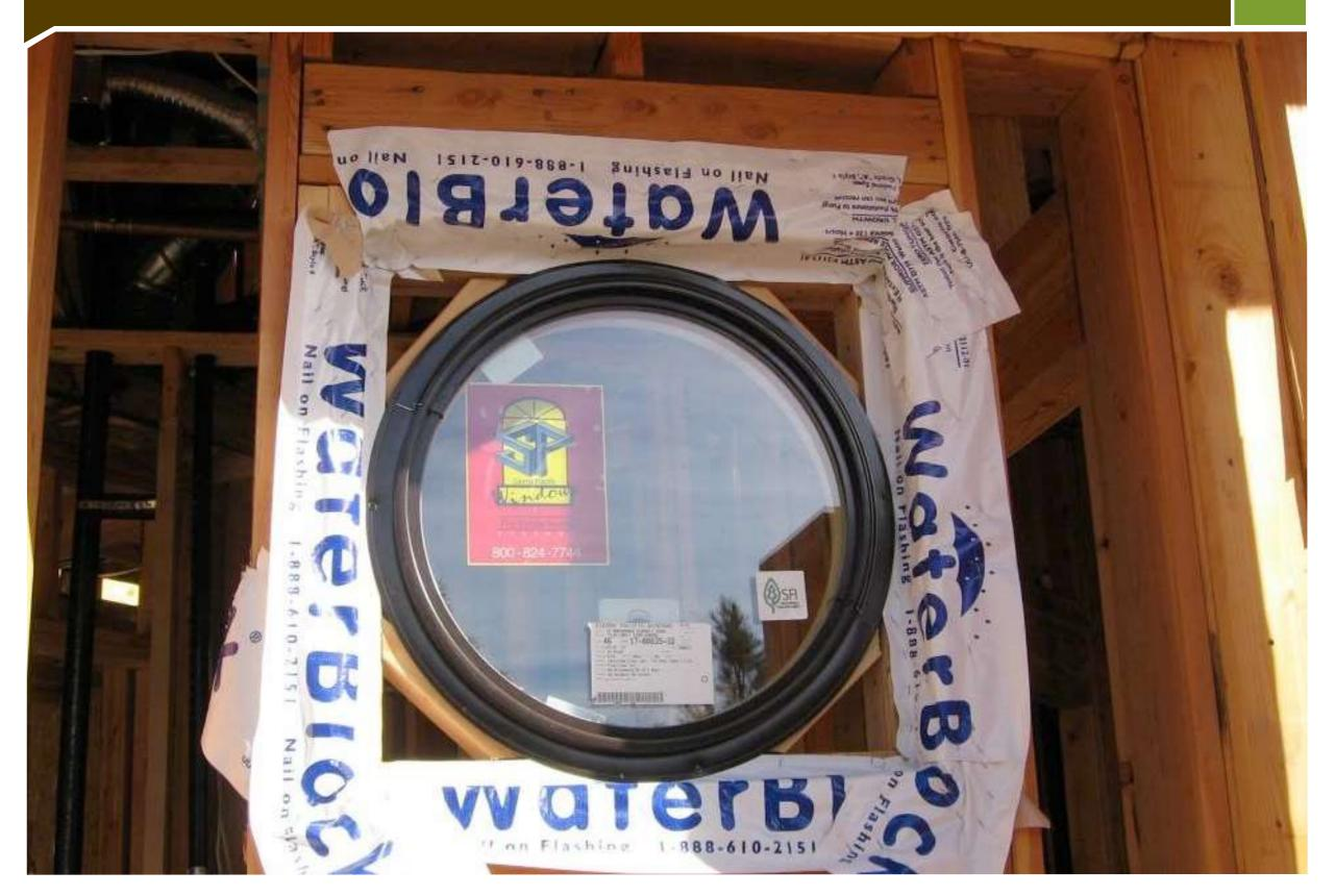
Site-Constructed or manufactured pan flashings for window and door openings in frame walls
