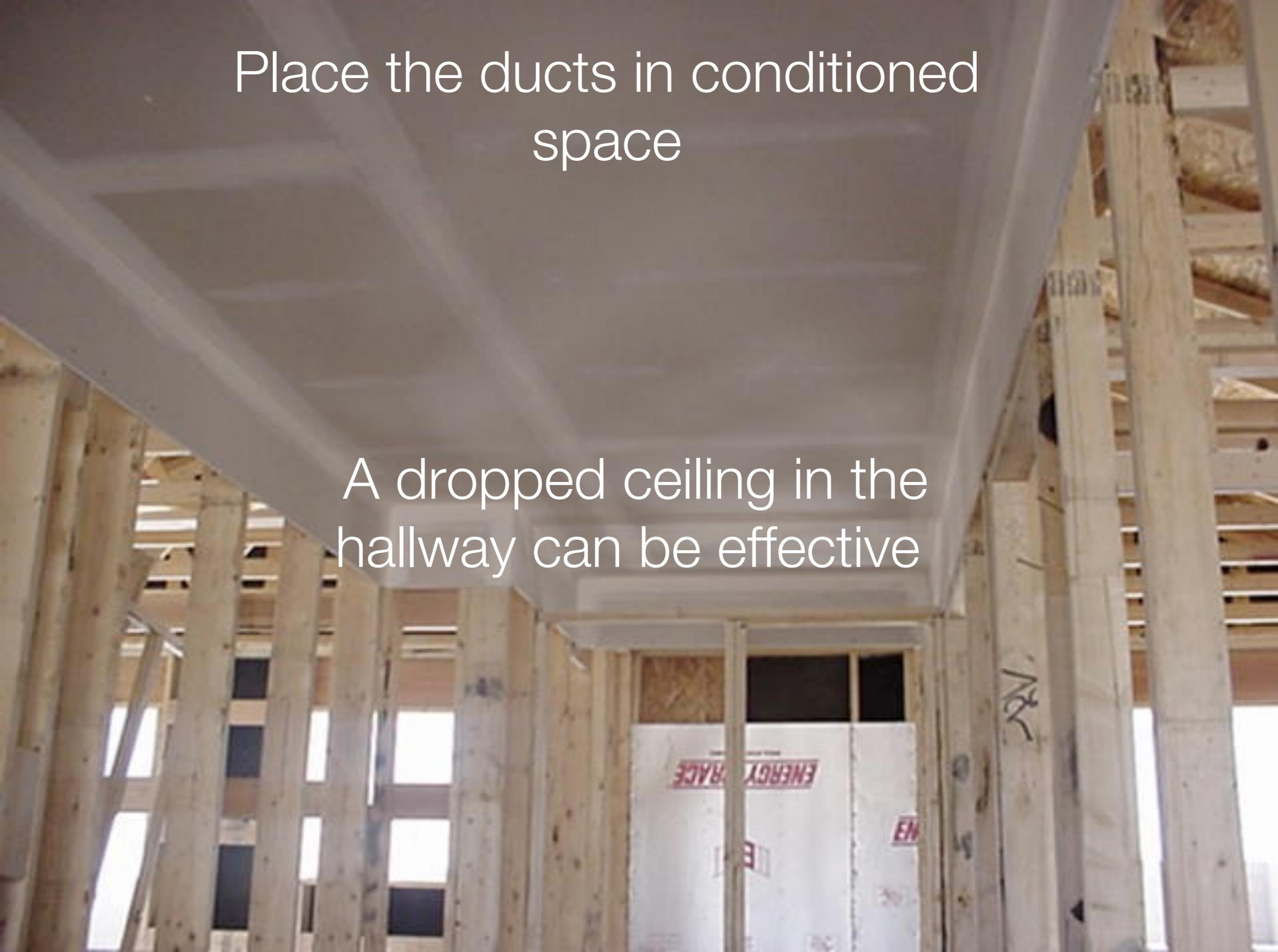
Ducts are now properly insulated and any duct leakage is to the interior
