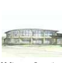
SCC Classroom Renovation and Addition
