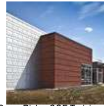
Camp Ripley COE Training Facility
