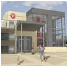
Maplewood Mall Parking Structure
