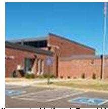
Minnesota National Guard Winona Armory Renovation
