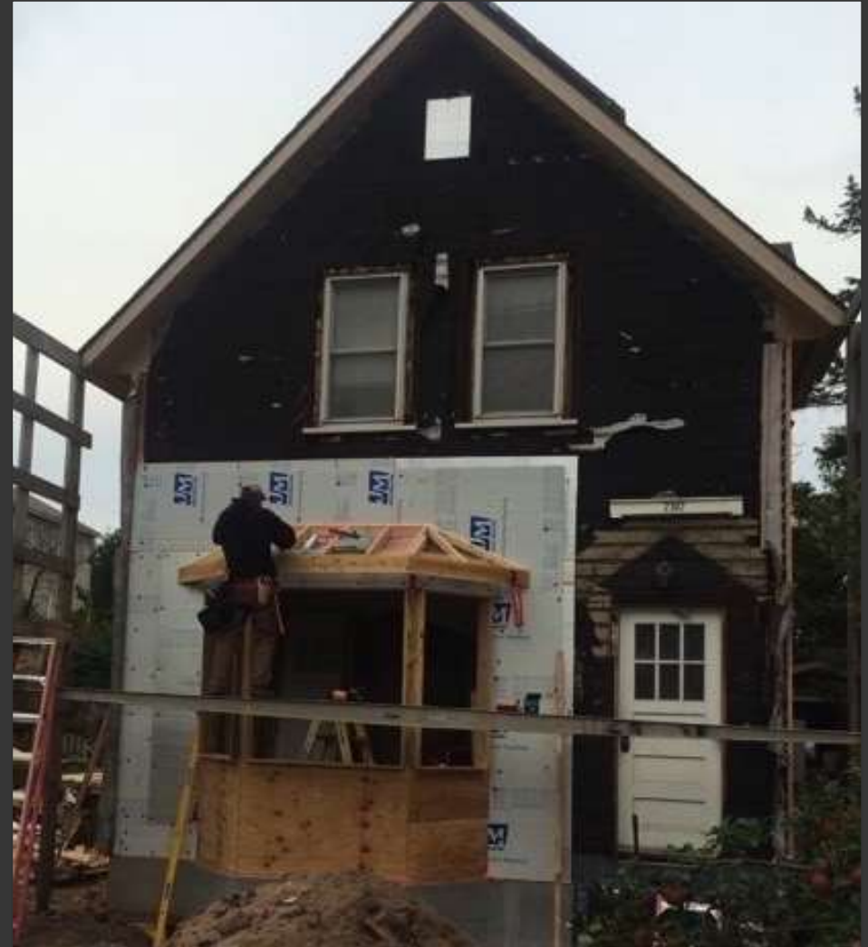
Retrofit with cellulose, rigid polyisocyanurate foam and closed cell spray foam.
