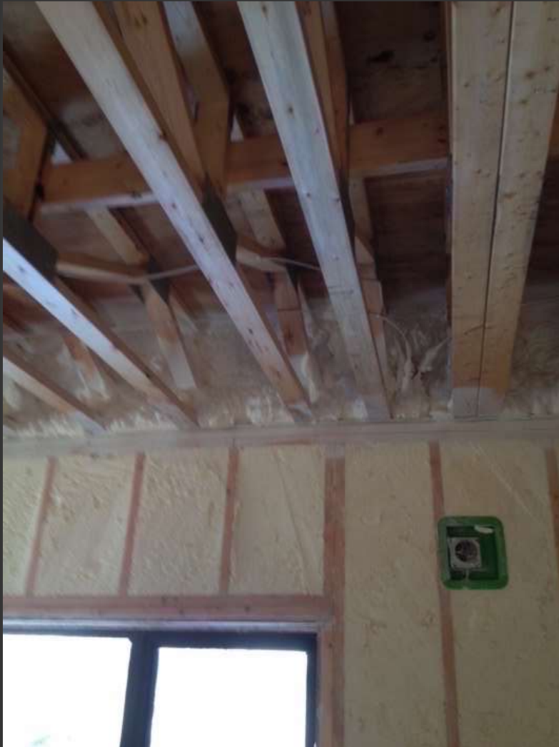
New Home with cellulose, open and closed cell spray foam.
