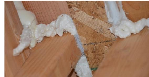
*Seal formed between gap in foam*
