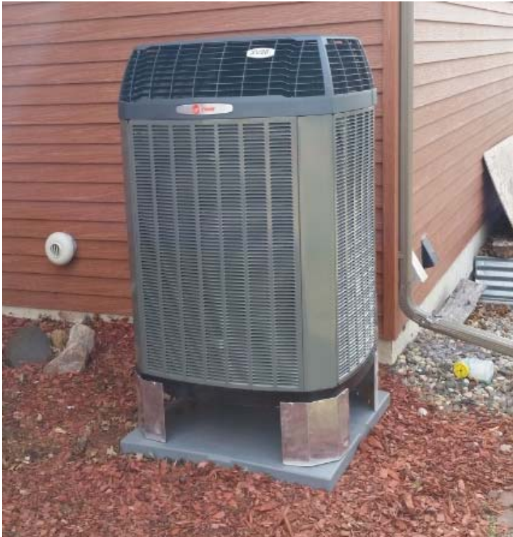
Ducted Whole-House Installation, Dual Fuel
