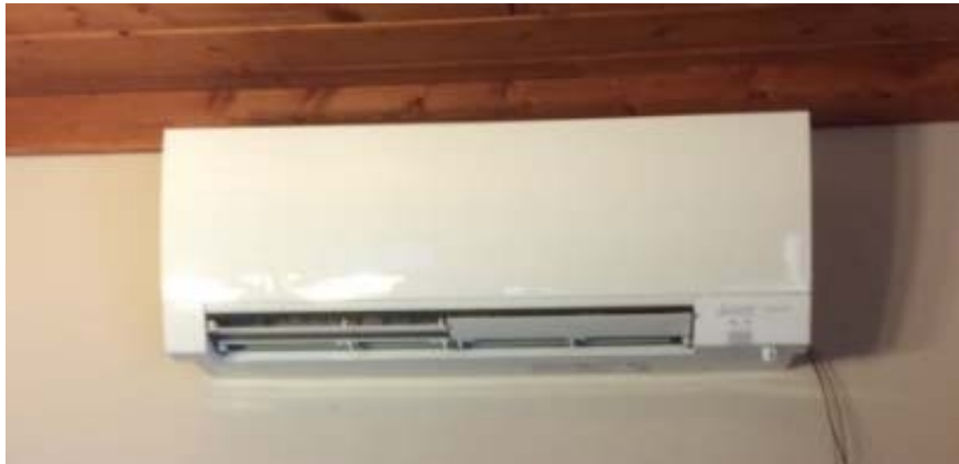
Ductless / Mini-Split Installation
