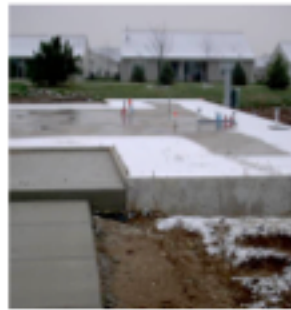
Slab on Grade
