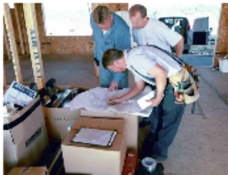
allowing a high performance building system installation in field
