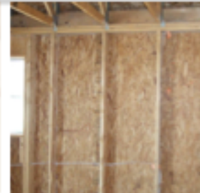
Reduce thermal bridges - reduce framing
