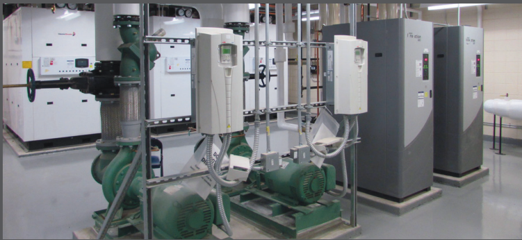
(Above) Variable frequency drives (white boxes over green motors) adjust speed depending on demand for heat. They slow down when there is not a lot of demand and speed up on cold days. (Right) The gymnasium is illuminated with LED lighting and lighting controls.
