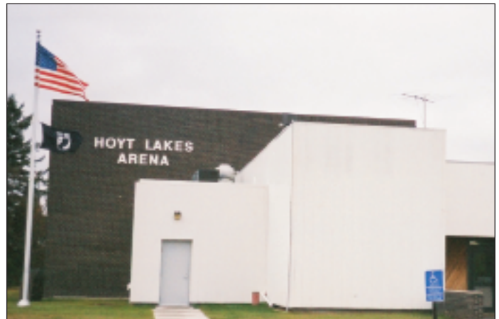
Recent conservation improvements to the Hoyt Lakes Arena earned a $5,819 PowerGrant Rebate from Minnesota Power.
