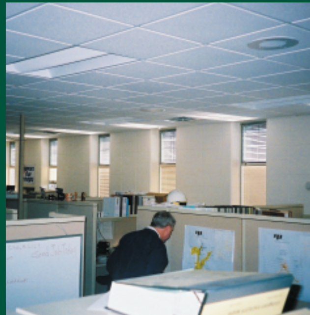
The upper sections of east-facing exterior windows are fitted with LightLowers™. They reflect incoming light off the ceiling so it reaches deeper into rooms.
