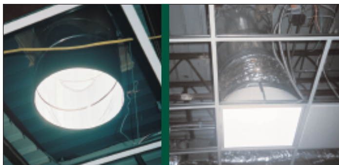
Prior to ceiling tile installation, it is easy to see how Vellux Sun Tunnel™ skylights draw natural light from the roof into windowless interior rooms using reflective tubes.
