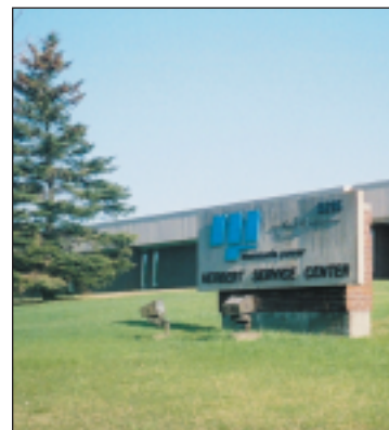
MP's newly remodeled Herbert Service Center in Duluth is a demonstration site for energy efficient technologies.
