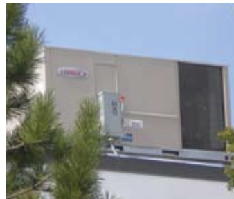
New energy-efficient air conditioning units and economizers are saving Minnesota Discovery Center nearly $5,000 in annual electric costs, providing comfort in public places, and maintaining climate conditions necessary for valuable library, archive and exhibit collections.
