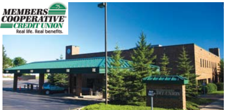
MCCU's Cloquet branch has switched to energy-efficient lighting.
