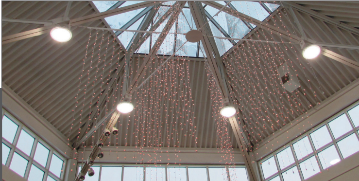
New LED lighting and other energy conservation upgrades enhance the experience for shoppers and retailers while saving Miller Hill Mall around 900,000 kWh and $55,000 per year.
