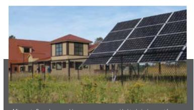
Minnesota Power's renewable energy program provided technical support for an onsite 40 kW solar photovoltaic system that meets 20-25 percent of the facility's energy needs.
