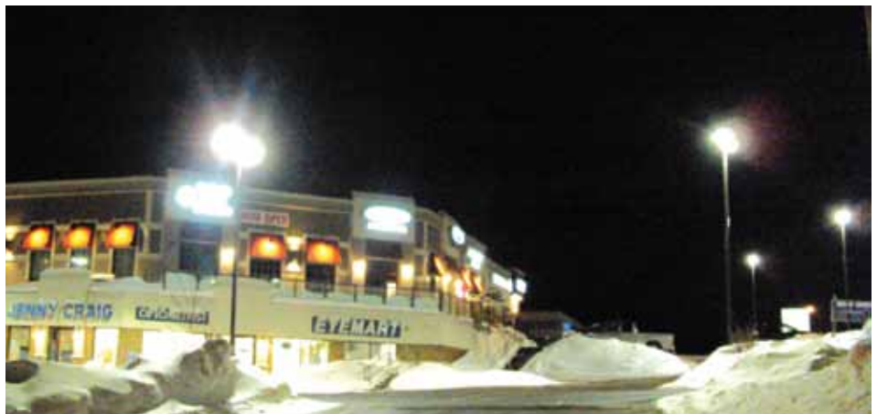
LEDs operate well at low temperatures, making them an ideal outdoor lighting choice in winter climates.
