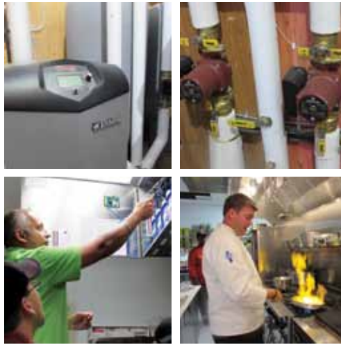
Top Row: The restaurant's mechanical systems are designed for energy efficiency. Bottom Row: Tanuj Gulati of Energy Insight, Inc. checks out the controls for the kitchen ventilation system. The exhaust system over the stoves have heat and smoke detectors and run only when needed.
