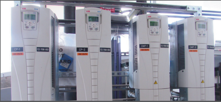
(Above) Variable frequency drives in UMD's Campus Utility Building adjust speed depending on cooling demand so pumps and fans do not have to run continuously at high speeds. (Right) UMD Sustainability Director Mindy Granley, Minnesota Power Business Services Advisor Craig Kedrowski, Minnesota Power CIP Consultant Tanuj Gulati, and UMD Facilities Operations Manager John Sawyer meet regularly to discuss energy efficiency.
