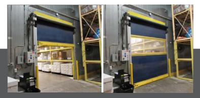
High speed automatic doors on coolers and freezers keep cold air from escaping, resulting in significant energy savings.
