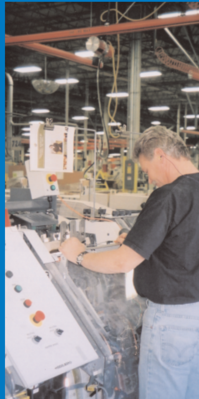
High-bay, T-8 fluorescent lighting in the bindery provides consistent, color-correct lighting, while saving energy.
