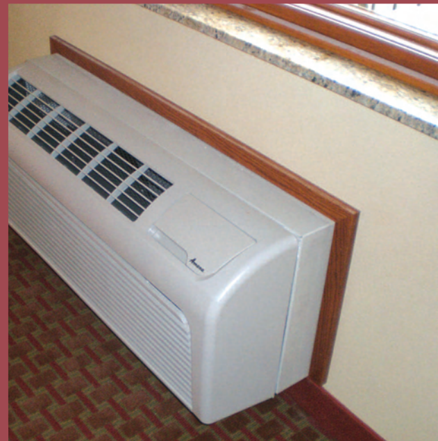
(Top) Energy-efficient, pulse-start metal halide parking lot lights hold their lumens over time and are fully shielded to prevent polluting the night sky or wasting energy. (Bottom) Individual PTACs allow room-by-room heating and cooling control. These units use 300 to 400 times less electricity and are much less expensive to install than baseboard or electric resistant heat.
