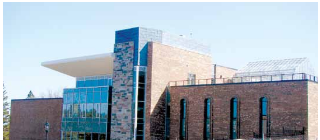
The new Science Center expansion at The College of St. Scholastica is a model of energy efficiency. Minnesota Power helped the design team identify energy- and cost-saving measures and provided funds for enhanced commissioning of the facility.
