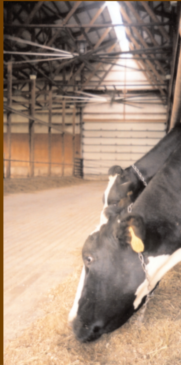
Enormous overhead fans powered by a VFD motor efficiently circulate air and keep cows at Oak Hill Dairy comfortable while eating.
