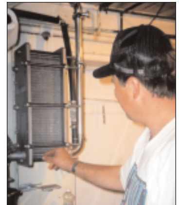
Larry Capko of Oak Hill Dairy explains an energy efficient plate cooler that chills milk using well water drawn from the ground.
