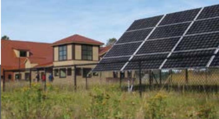
Minnesota Power’s renewable energy program provided technical support for an onsite 40 kW solar photovoltaic system that meets 20-25 percent of the facility’s energy needs.
