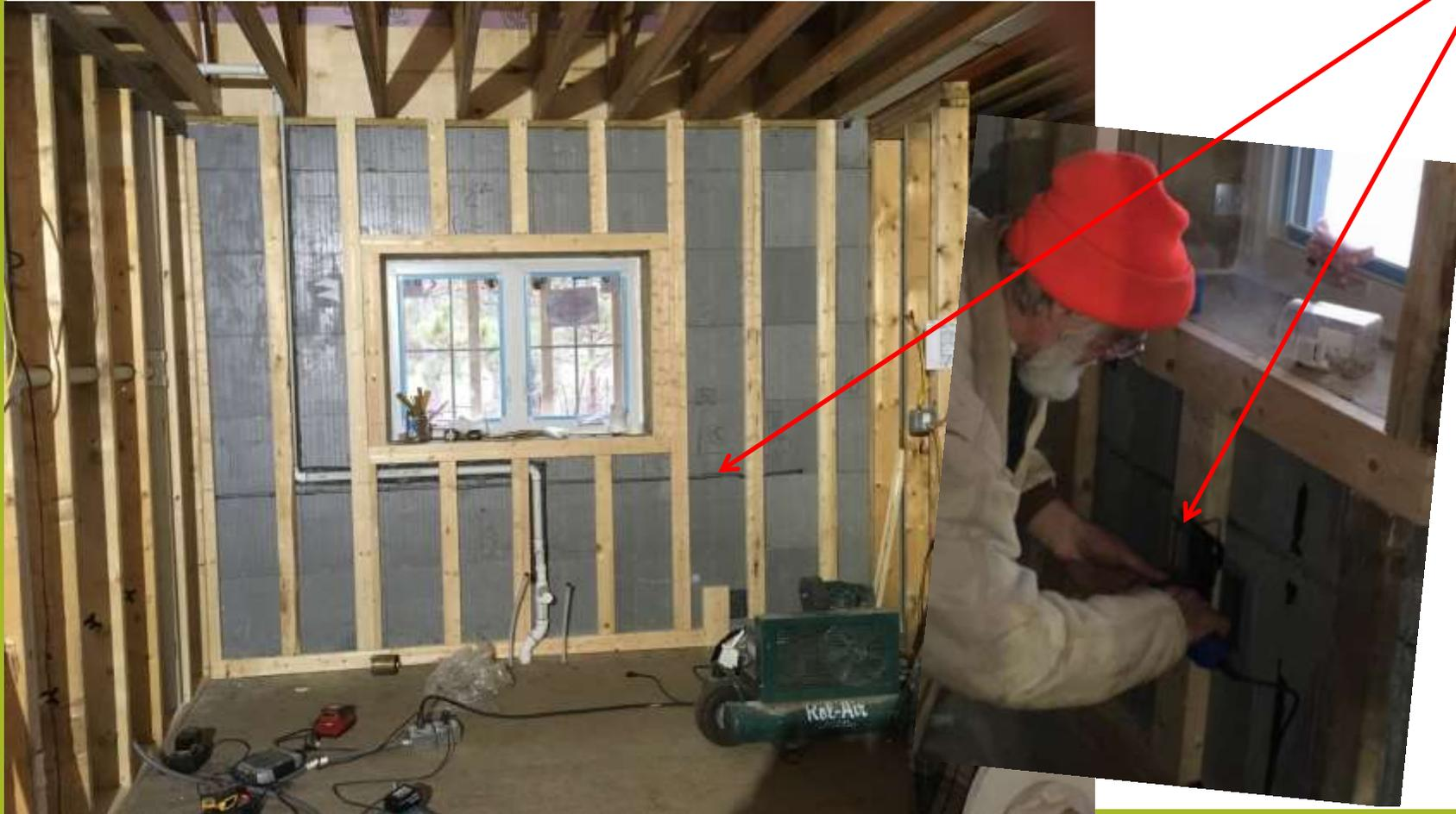
Less room on the main floor to run electrical & plumbing on outside walls. We used a hot knife to cut the ICF foam, installed the electrical & plumbing then foamed over it.
