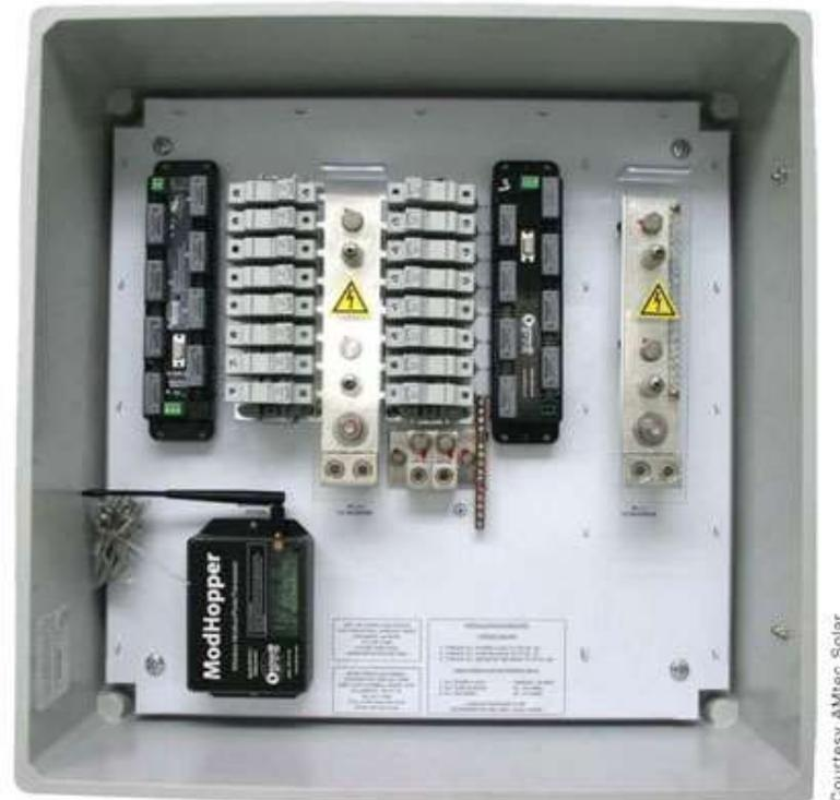
String-level granularity - This Prominence series smart combiner from AMtec Solar provides string-level monitoring for 16 source circuits and includes an optional wireless Modhopper.
