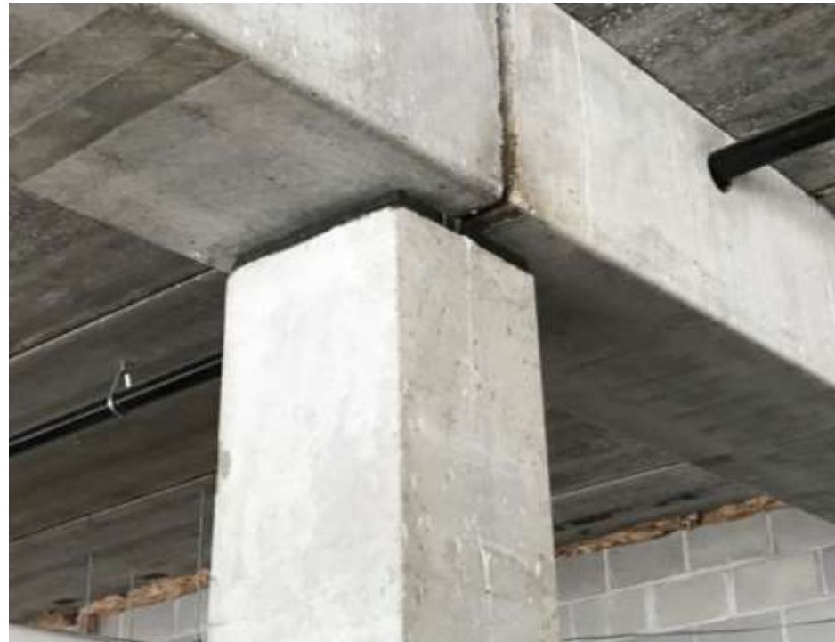
THERMAL BREAK AT TUCK-UNDER PARKING
