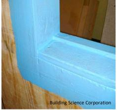
Photograph 11: Window Opening—Origami is not a necessary skill with fluid applied flashing systems.
