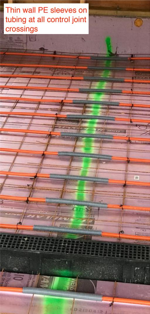
Thin wall PE sleeves on tubing at all control joint crossings
