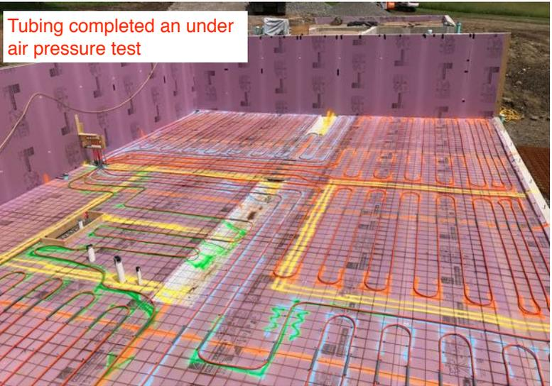
Tubing completed an under air pressure test
