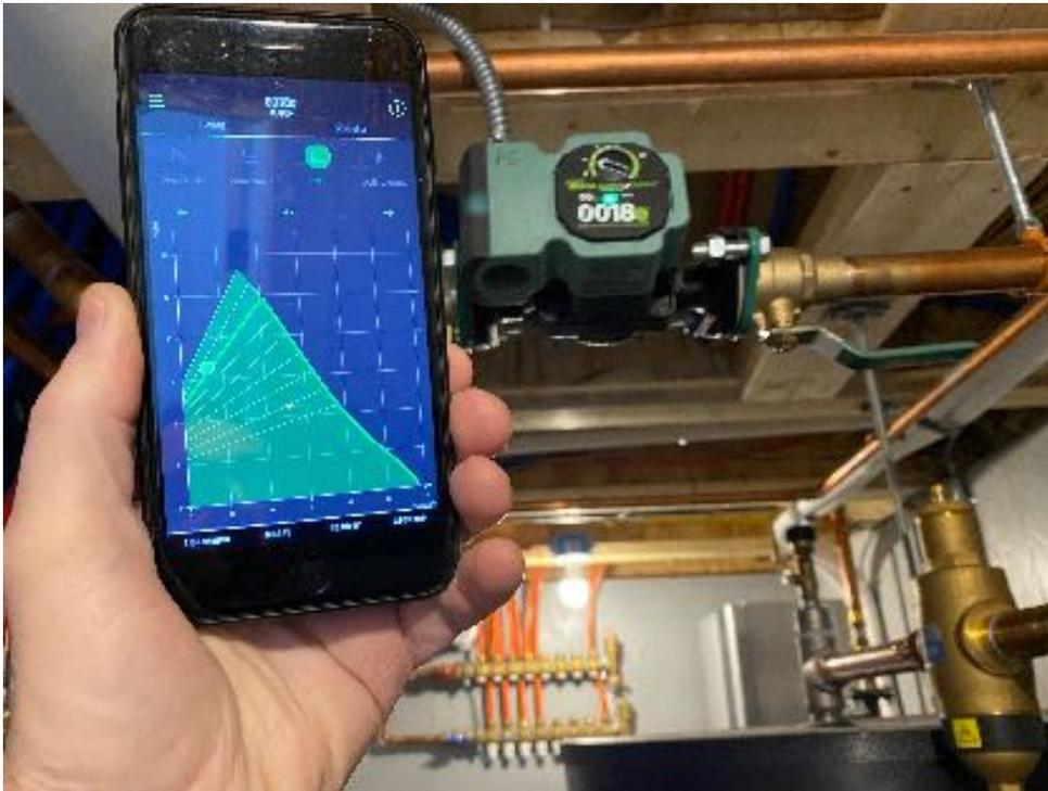
The Taco0018e circulator serving main floor operates continuously whenever system master switch is set to heating. It can operate in either proportional or constant differential pressure mode.
