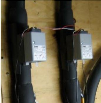
• Don't insulate zone valve actuators or circulator motors (they need to dissipate heat)
