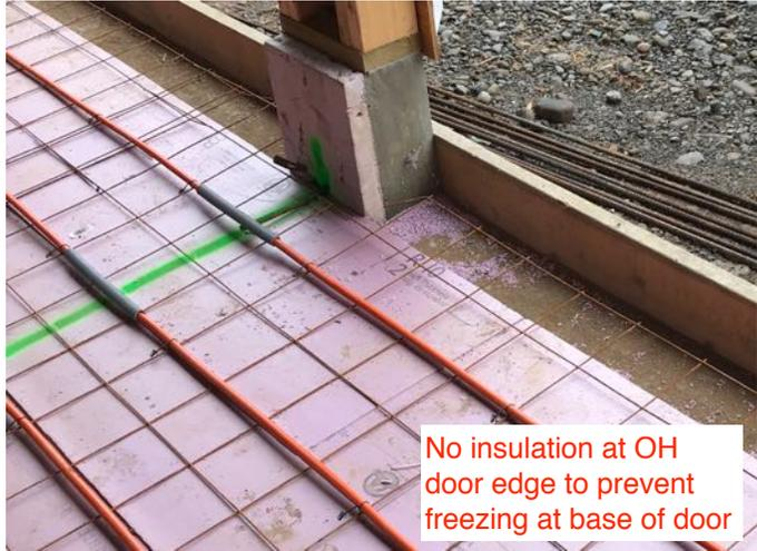
No insulation at OH door edge to prevent freezing at base of door
