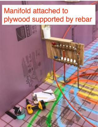
Manifold attached to plywood supported by rebar
