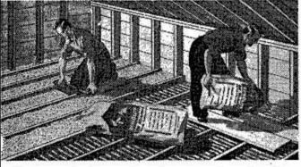
Plan now to insulate your home for year-round comfort with safe, fireproof Zonolite. Be as much as 15 degrees cooler indoors in summer. Save up to 40% on fuel in winter. You can do the job yourself with Zonolite. Simply pours into place between joists in attic and studs in sidewalls.
