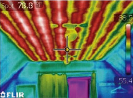
Thermal image of radiant ceiling in operation
