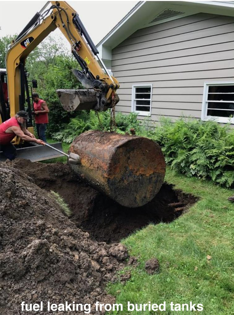
fuel leaking from buried tanks
