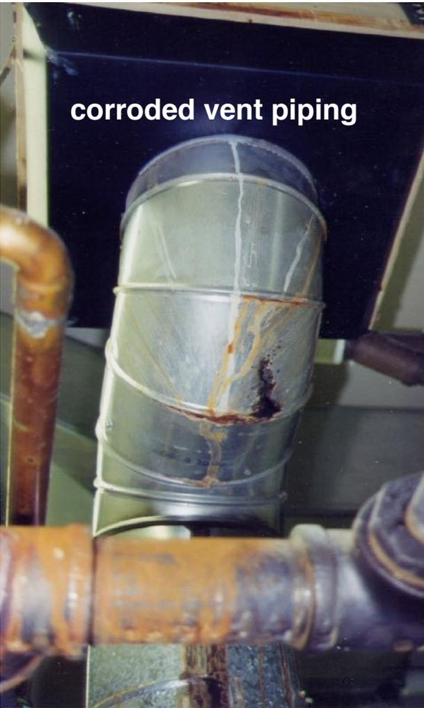
corroded vent piping
