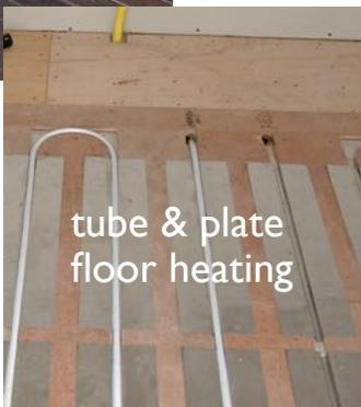
tube & plate floor heating
