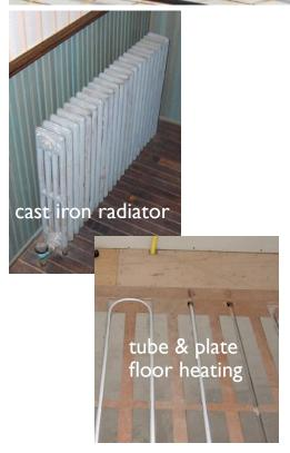
A comparison of THERMAL MASS for several heat emitters: All heat emitters sized to provide 1000 Btu/hr at 110 °F average water temperature, and 70 °F room temperature:
