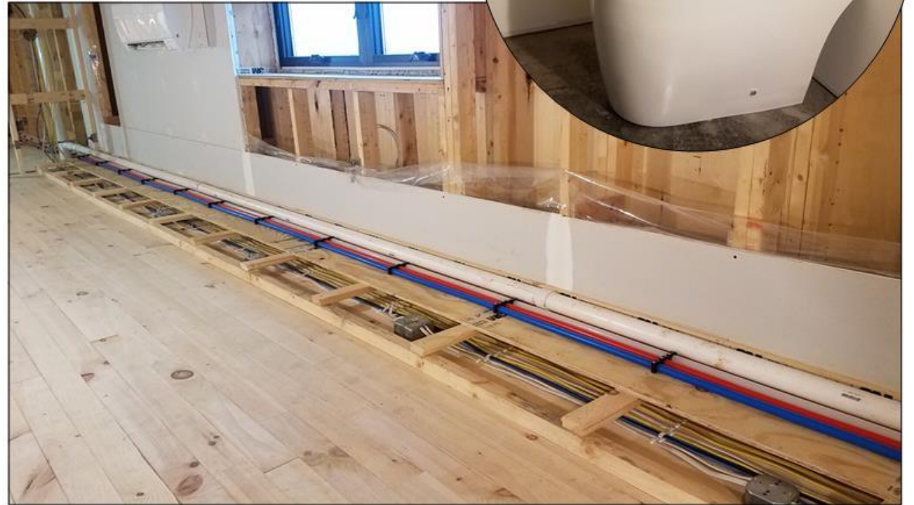
Plumbing + Wiring Chase
