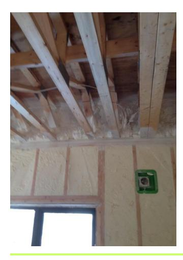
Cavity insulation is often integrated into structure. How and how often will it be disrupted?
