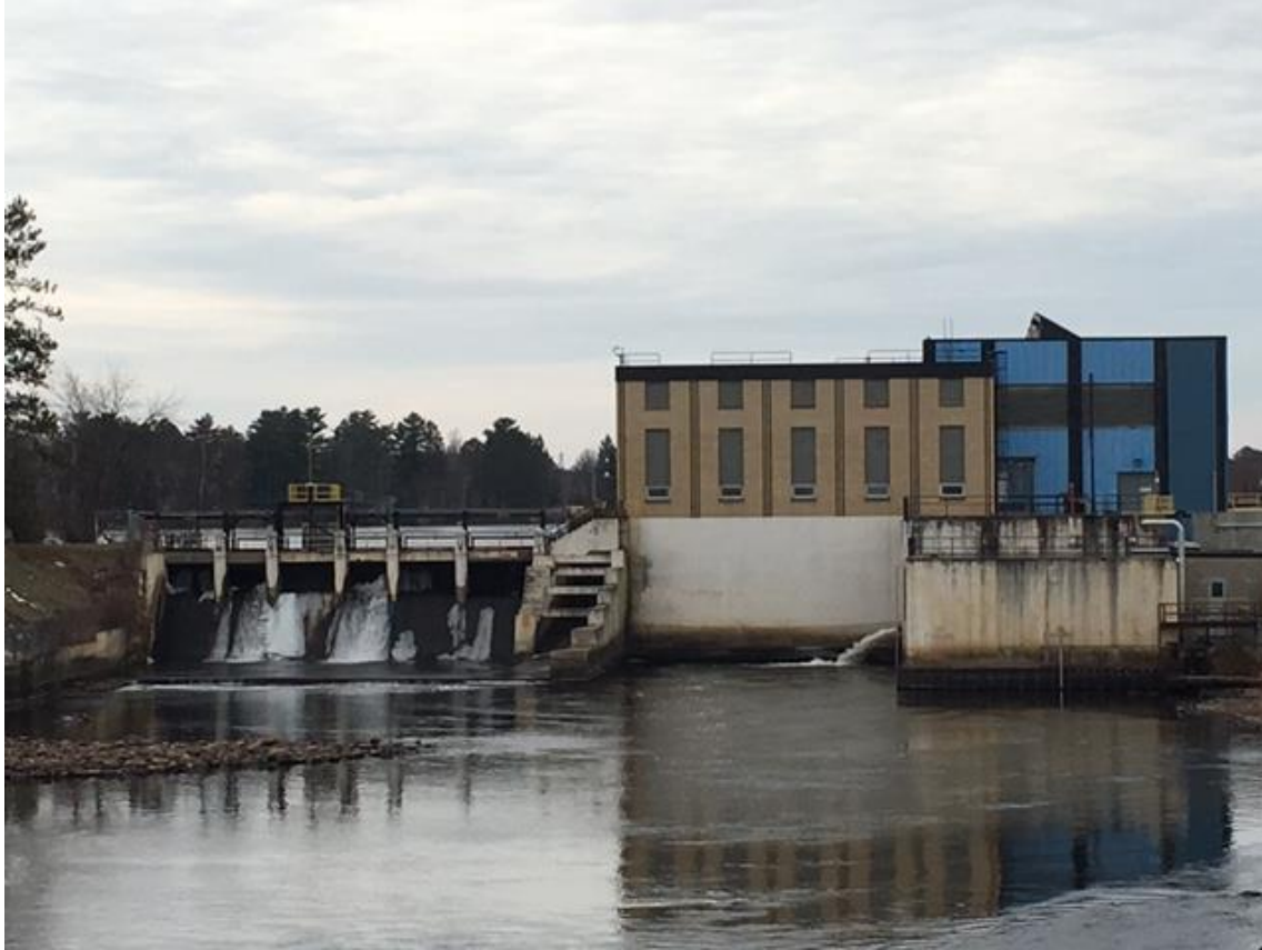
Photo E.10-2 Grand Rapids Project powerhouse
