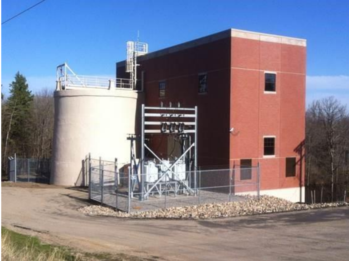
Photo E.10-4 Prairie River Project powerhouse
