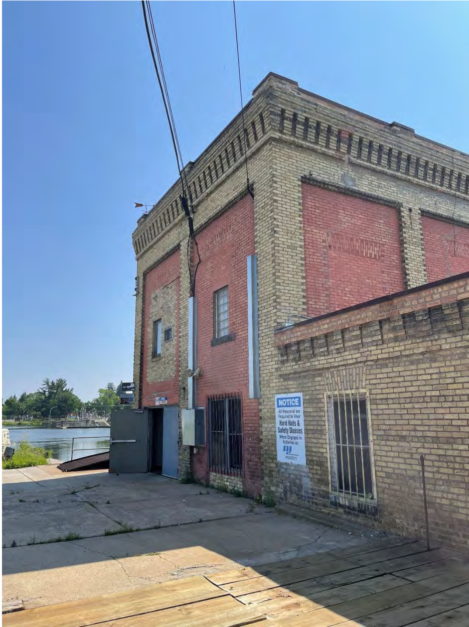
Photo 4-33: Little Falls Project Powerhouse Units 5 and 6
