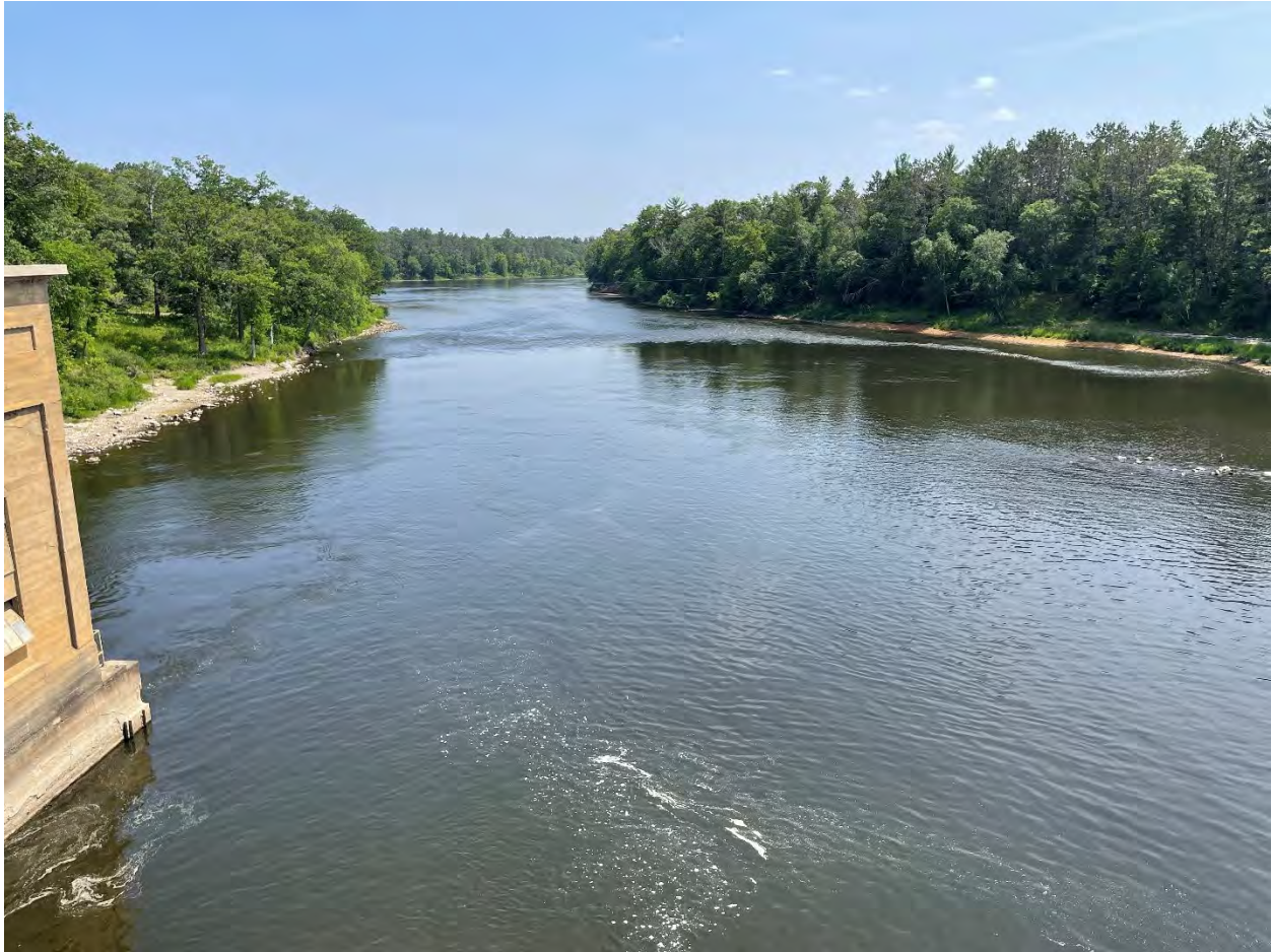
Photo 4-38: Sylvan Project Tailwater View from Spillway
