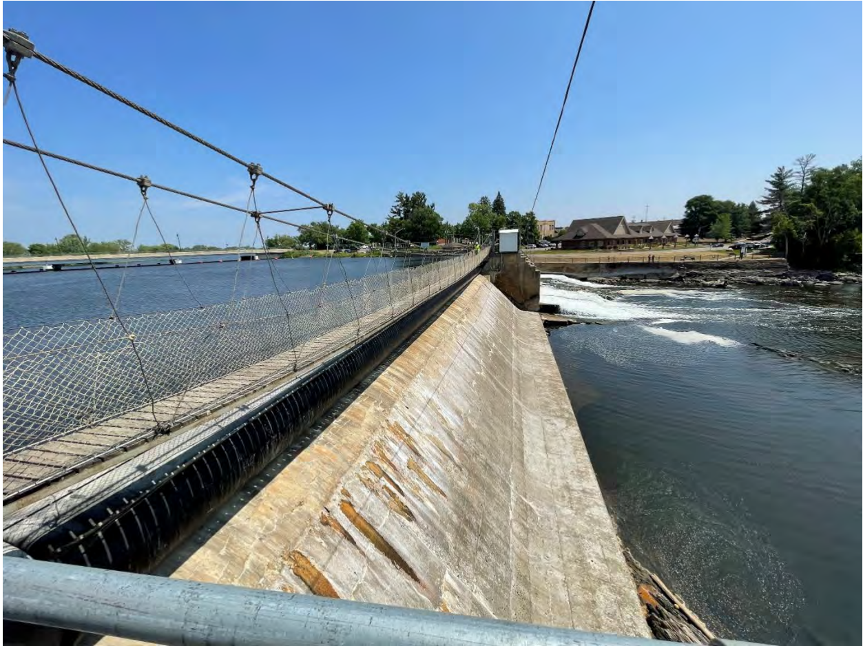
Photo 4-29: Little Falls Project Spillway Facing East
