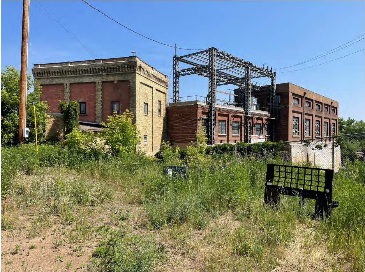
Photo 4-32: Little Falls Project Powerhouses
