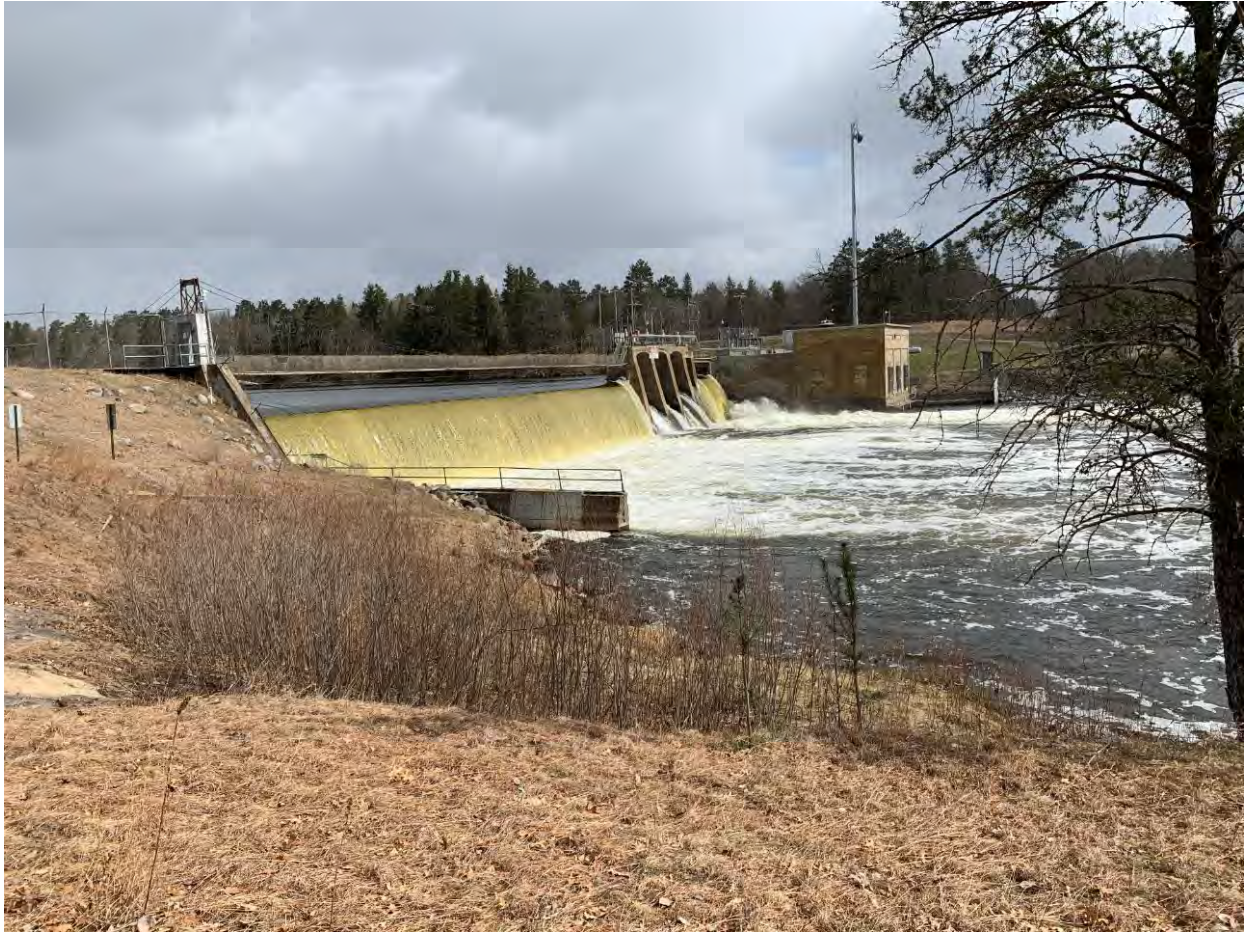
Photo 4-36: View of Sylvan Project Dam
