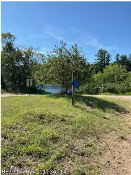
Date: 2024-08-31 Location: 46.3255°, -94.4104° Description: Handicap parking signs, falling down
