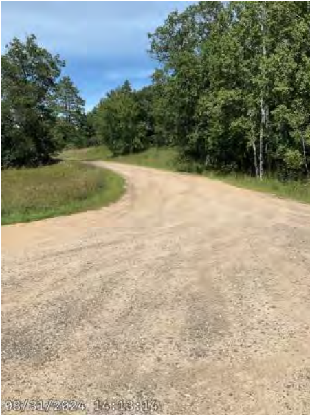
Date: 2024-08-31 Location: 46.3042°, -94.3760° Description: Access road above parking areas
