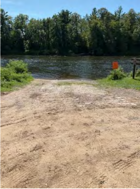
Date: 2024-08-31 Location: 46.3038°, -94.3763° Description: Boat launch Photo Type: BL
