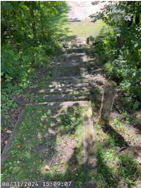
Date: 2024-08-31 Location: 46.3040°, -94.3759° Description: East parking lot stairs to boat launch. Photo Type: PT
