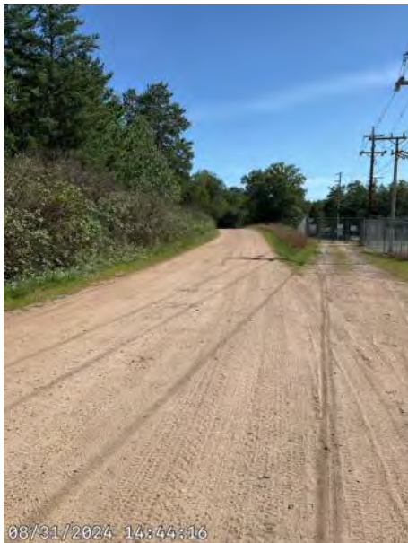
Date: 2024-12-19 Location: 46.3058°, -94.3773° Description: Access road
