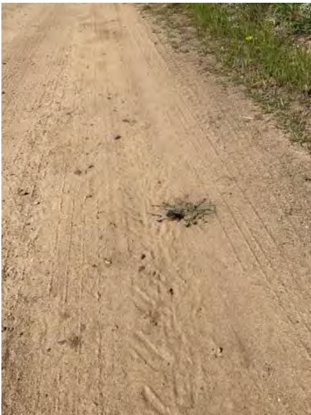
Date: 2024-12-19 Location: 46.3056°, -94.3772° Description: Rebar rod sticking out of the ground along the access road above substation
