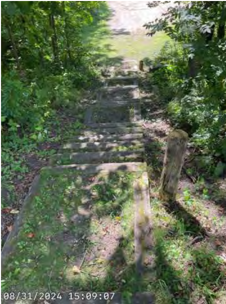
Date: 2024-12-19 Location: 46.3040°, -94.3759° Description: Stairs from parking area to boat launch
