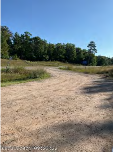
Date: 2024-08-31 Location: 46.3116°, -94.3805° Description: East parking lot access road
